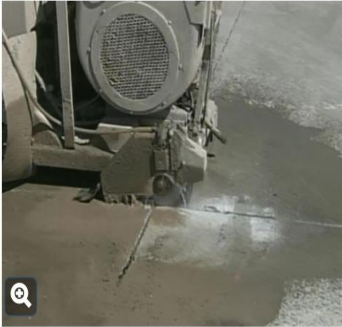
Sawing a Type B Repair
