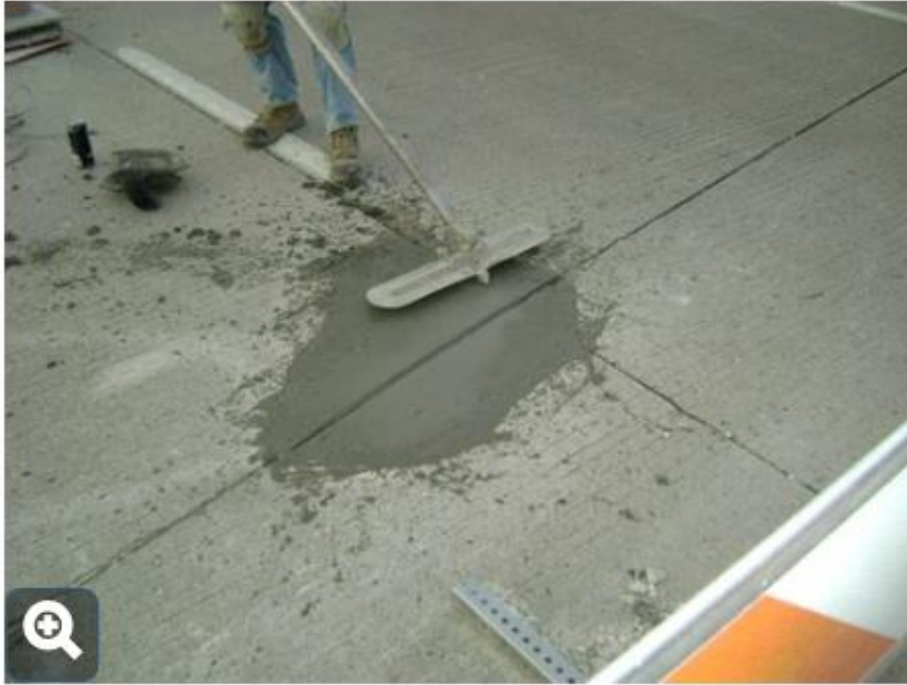
Tooling the joint in preparation for green sawing
