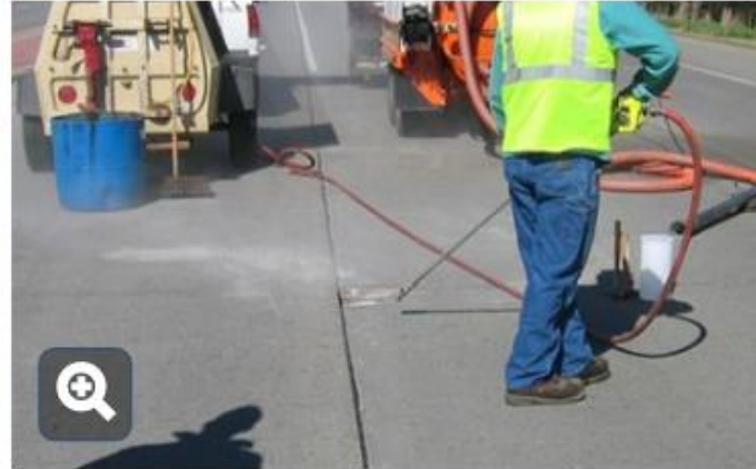
Maintenance crew using compressed air for final cleaning.
