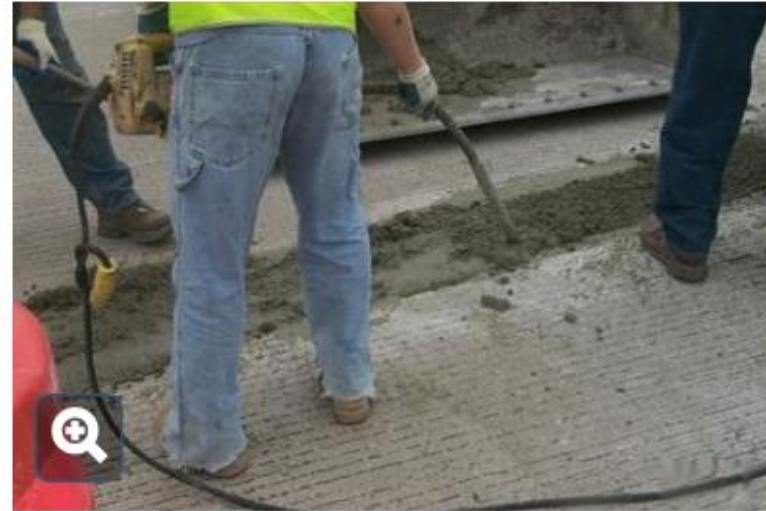
Vibrating 3U18 patching mix.
