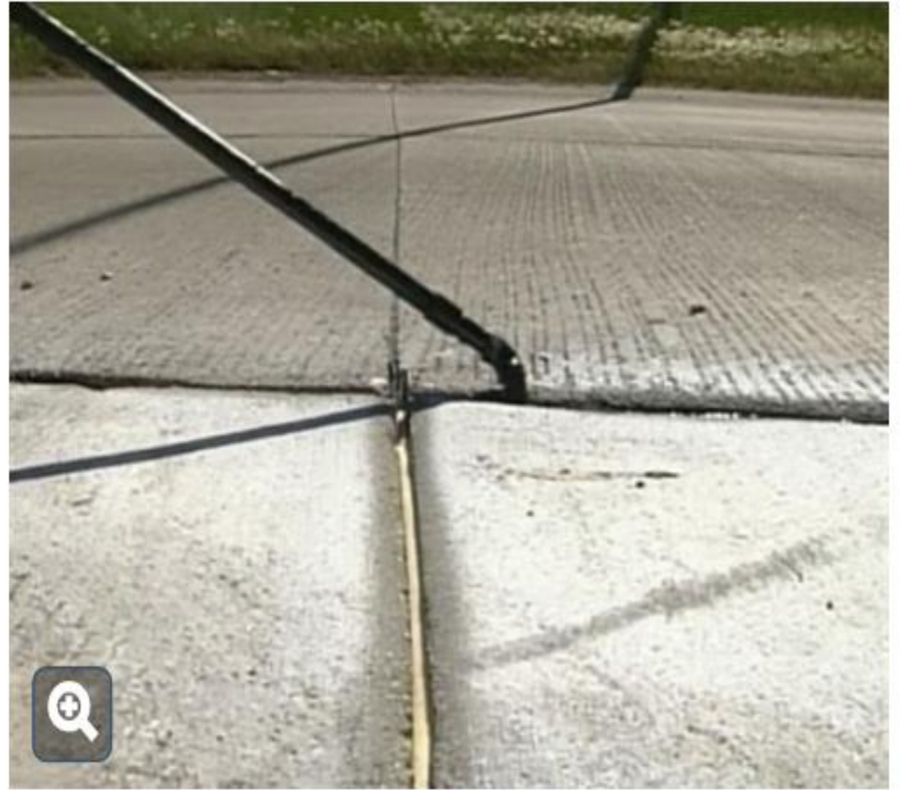
Sealing along a Type B repair
