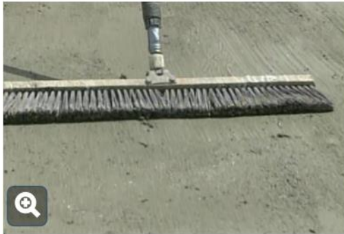
Broom texture for skid resistance
