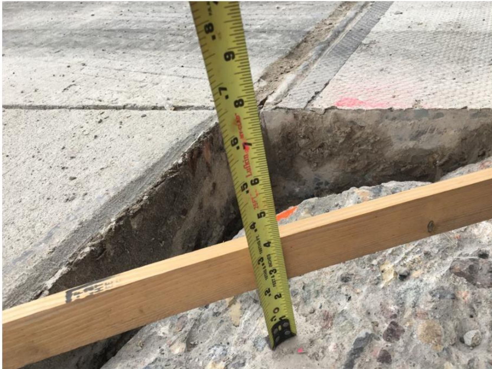
Using a straightedge (lath) to check partial depth repair is a minimum of 2" deep
