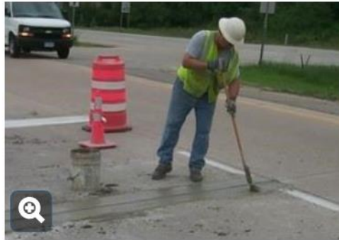
Applying sacrificial grout layer over tapered edges
