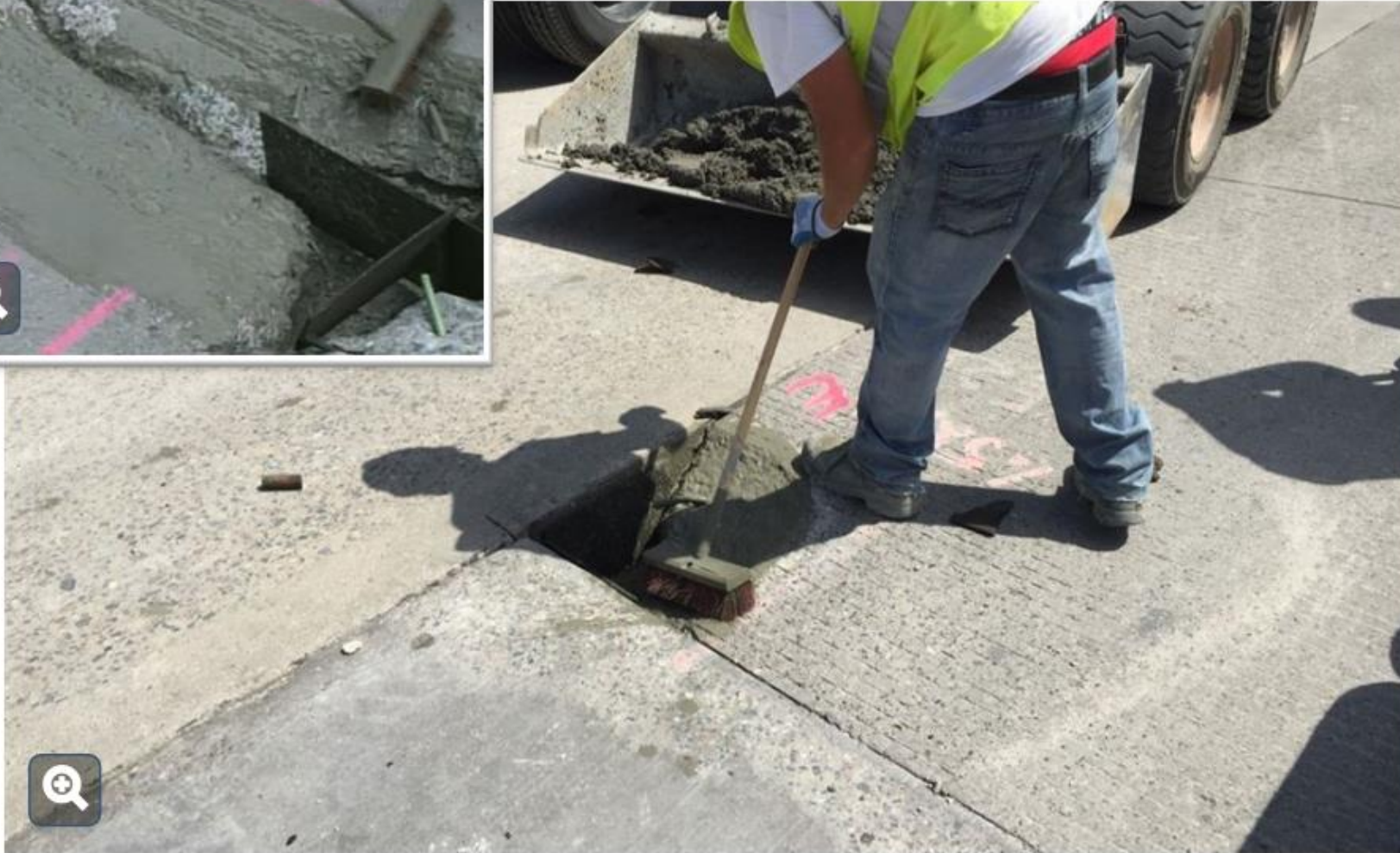
Applying bonding grout to the partial depth repair
