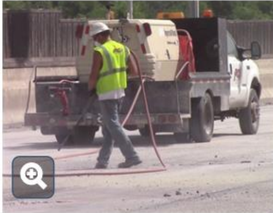
Compressed air blasting the repairs
