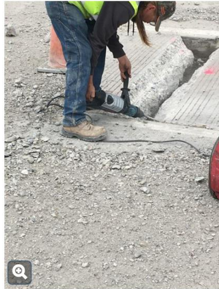
Drilling 1/8" oversized holes
