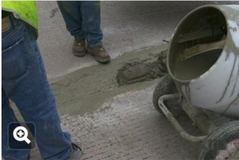
Placing 3U18 concrete patching mix just after applying bonding grout.
