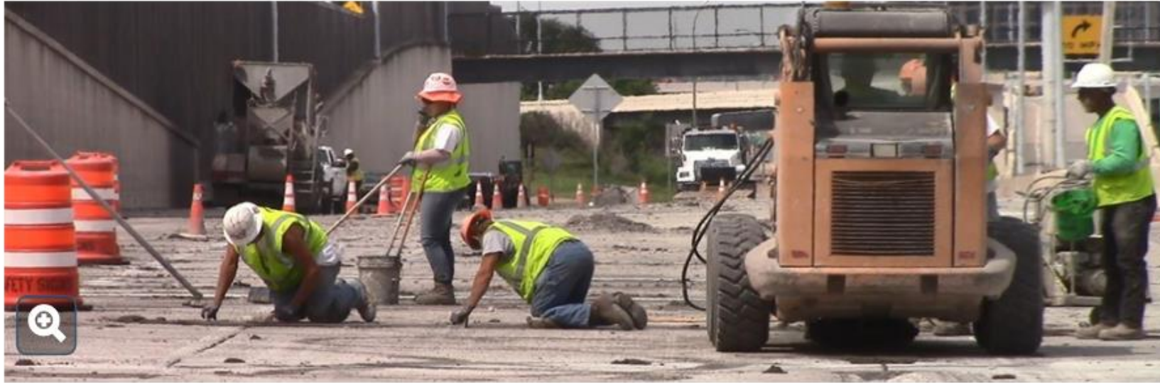
Finishing and edging partial depth repairs.
