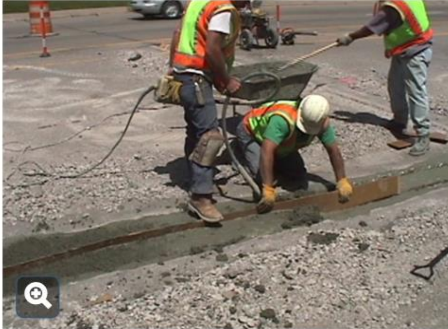
Re-establishing joint above random crack with wax coated cardboard.
